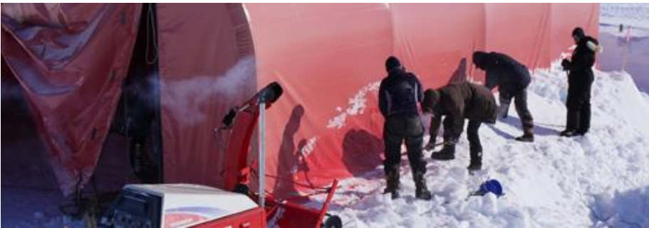
Cutting and hammering ice away from the garage.
